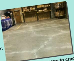
Conventional concrete prone to cracking.
